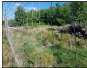
Wire stock fencing
